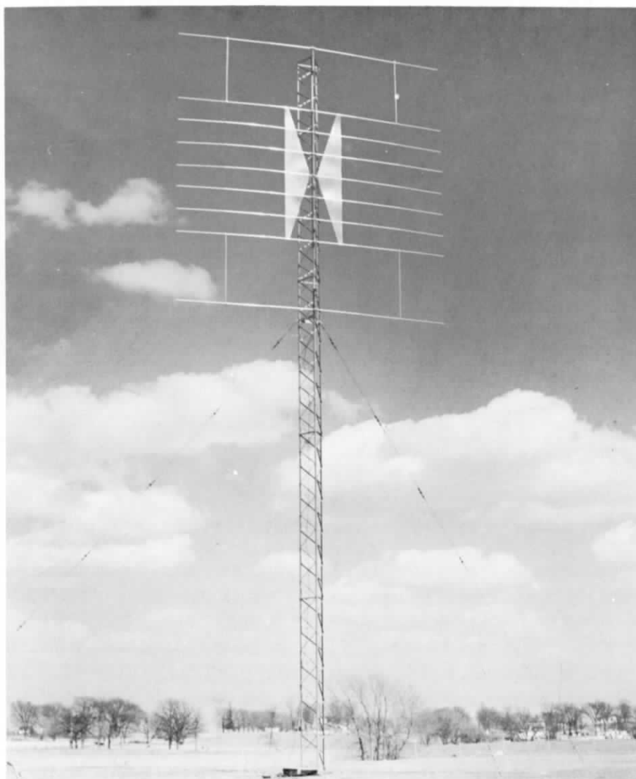
Figure 23. Typical Installation of a 10- to 25-mc Horizontally Polarized Broadband Dipole Antenna.
