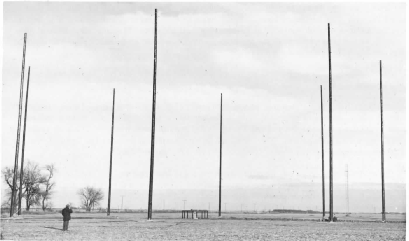
Figure 16. Typical Installation of a 2- to 11-mc Inverted Discone Antenna.
